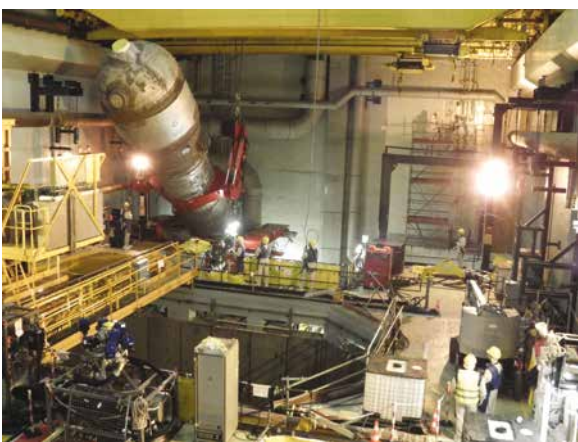
FIGURE 19 - EXTRACTING THE STEAM GENERATORS AT CHOOZ A
