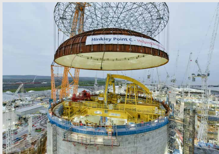
HPC – LIFTING THE DOME ONTO UNIT 1
